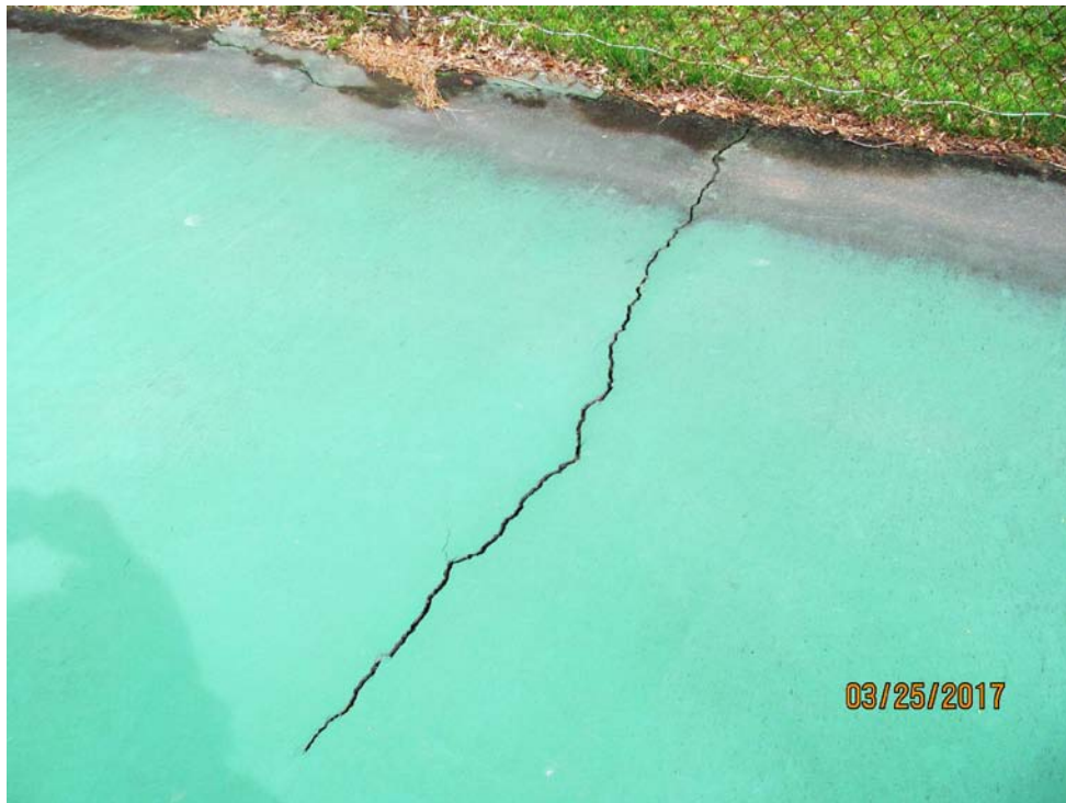
Photograph No. 32: Crack in tennis court deck.
