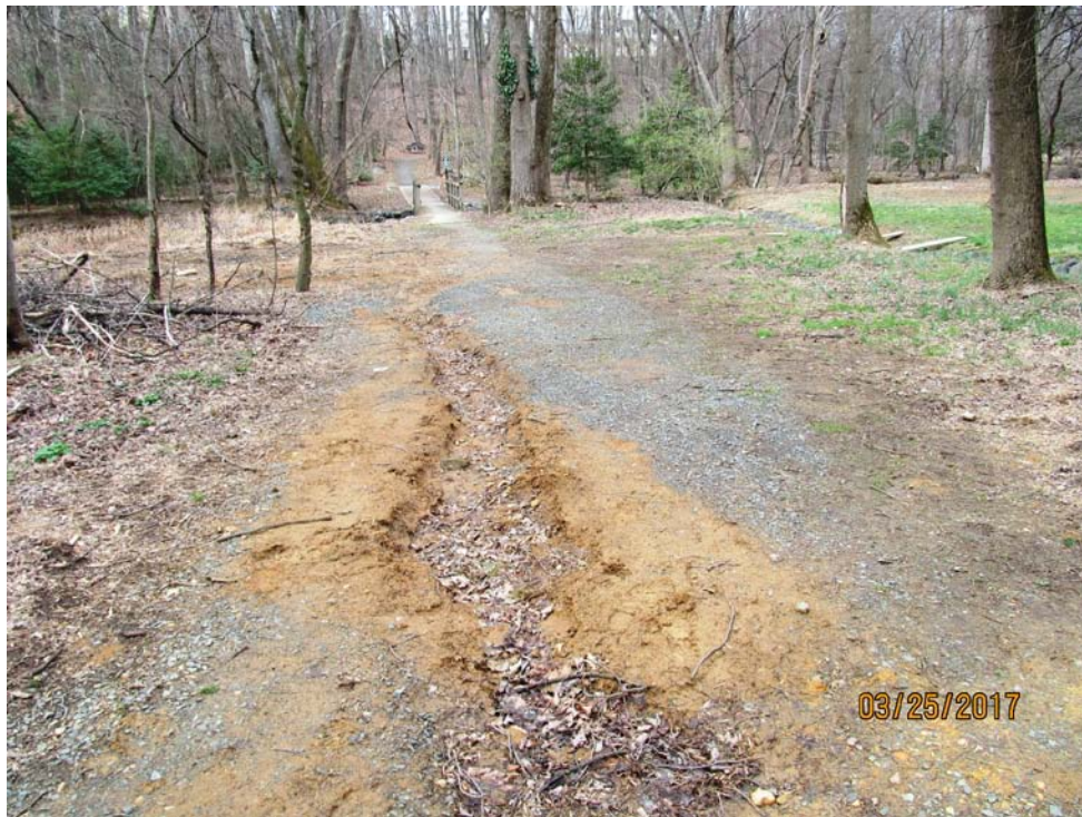
Photograph No. 44: Deteriorated trail at east end of Bridge #3.
