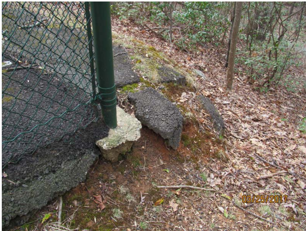
Photograph No. 13: Post footing erosion at All-Purpose Court.
