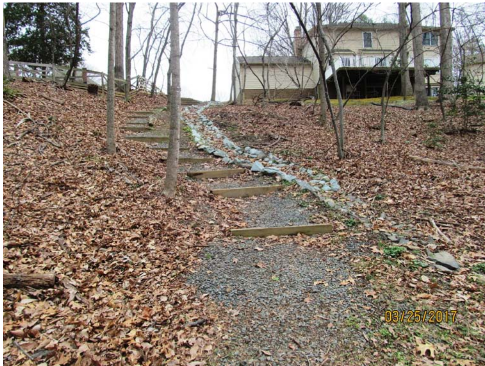
Photograph No. 48: Wood sleeper steps to Glenridge Court.
