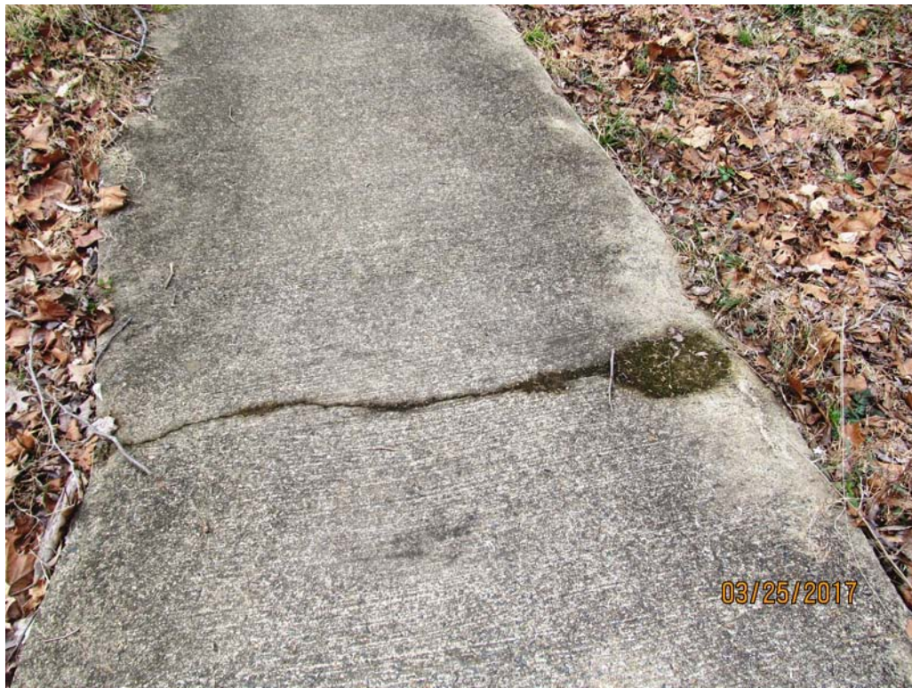
Photograph No. 19: Crack in concrete approach to Bridge #1.
