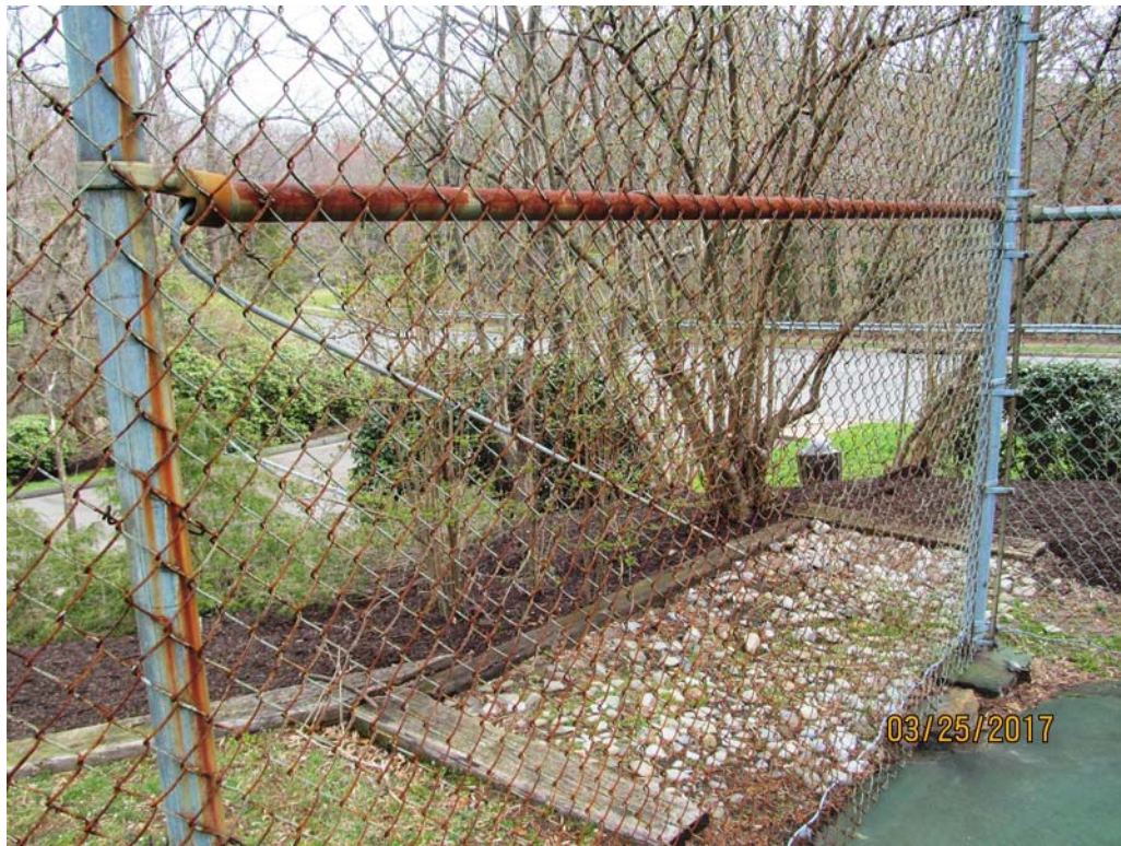
Photograph No. 33: Typical fence deterioration (corrosion) at tennis courts.
