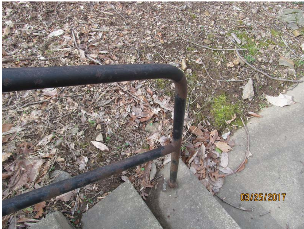
Photograph No. 5: Typical corrosion at step railings.
