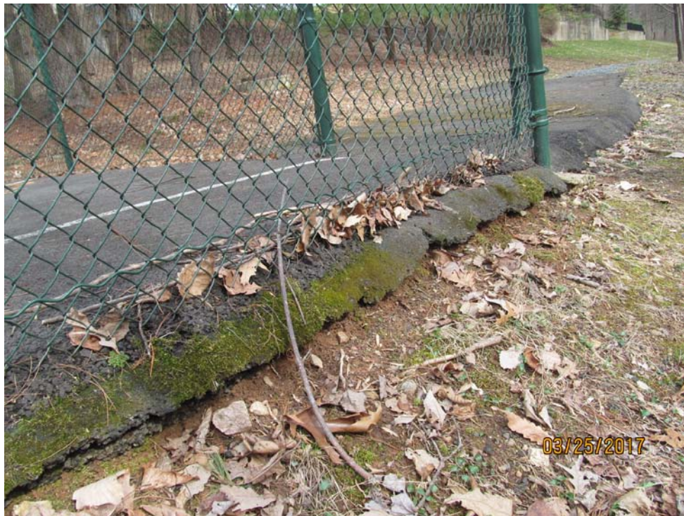
Photograph No. 14: Surface edge erosion at All-Purpose Court.
