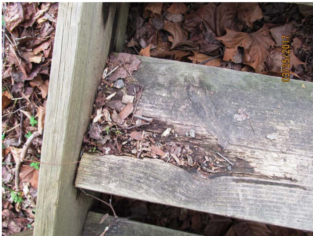
Photograph No. 21: Deterioration at wood steps.
