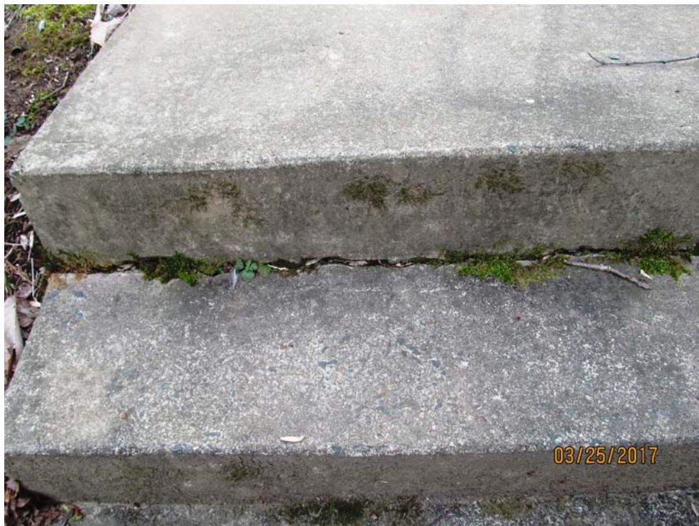
Photograph No. 6: Step crack.
