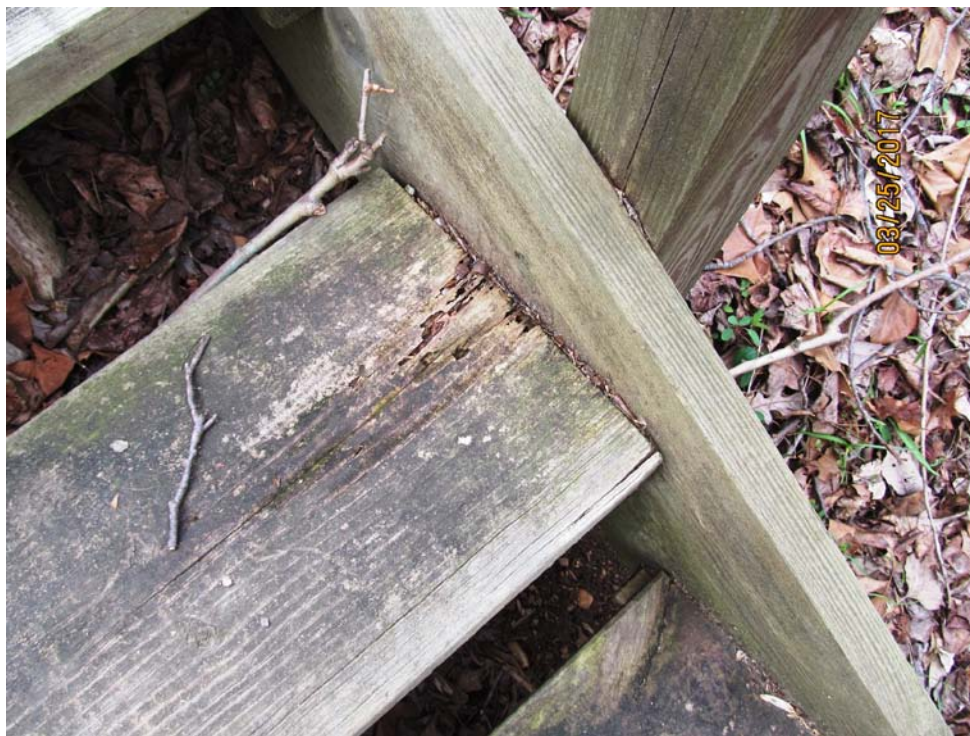
Photograph No. 22: Deterioration at wood steps.
